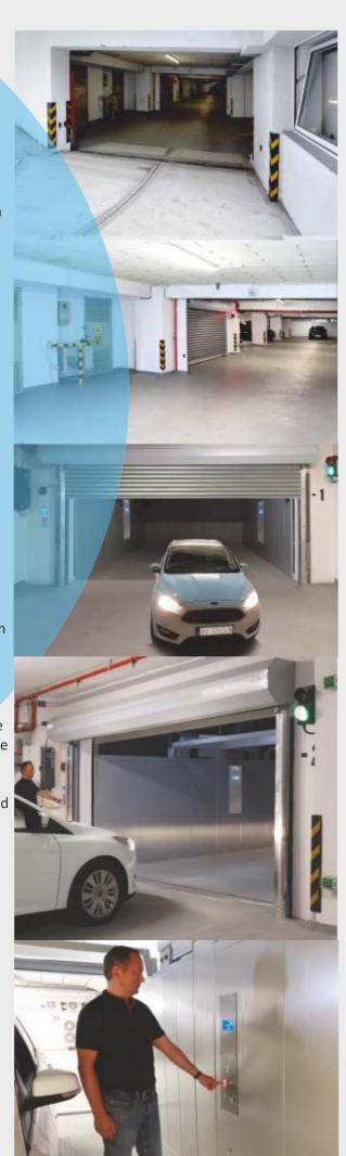
The safety light barriers ensure protection when entering and exiting the car lift.
